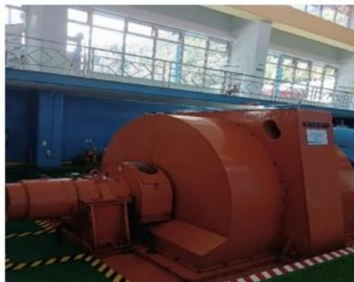
Gambar 1. 17 Generator PLTA Batang Agam
