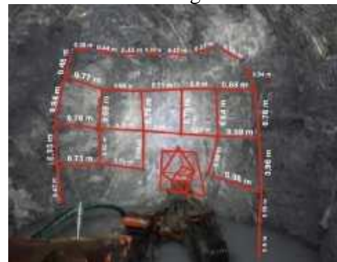
Figure1. Drilling Pattern Heading CKN_DC (16-02-2015)
