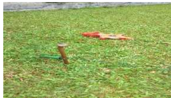
Figure 7. Grounding Resistivity Measurements in Building PTIPD UIN Suska Riau
