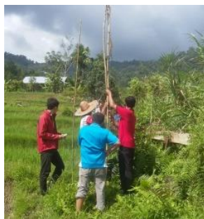
Fig. 3. Water head and piping system measurement
